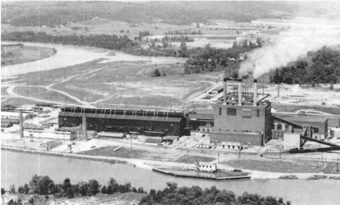
S-50 Liquid Thermal Diffusion Plant (long, dark building) The adjacent K-25 power plant shown with 3 smokestacks drew water from the Clinch River Clinton Engineer Works, 1945. Public domain (Courtesy of Barbara Scollin)
